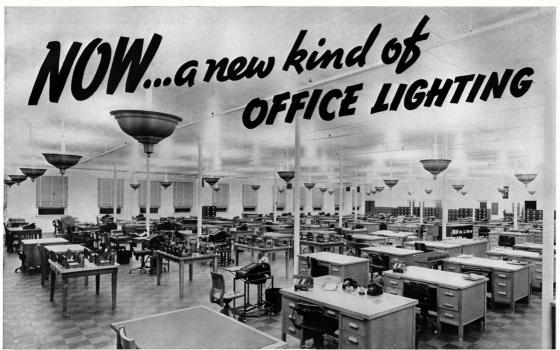
• The newest thing in office lighting is this combination of mercury and incandescent lamps in the general office of the Cannon Mills at Kannapolis, N. C. Each of the totally indirect luminaires contains one 400-watt mercury lamp and four 200-watt MAZDA lamps. Illumination of about 30 footcandles is provided.
